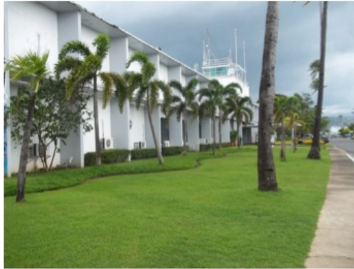
Figure 3: Adaption of Military Buildings—Subic Bay Metropolitan Authority Headquarters
