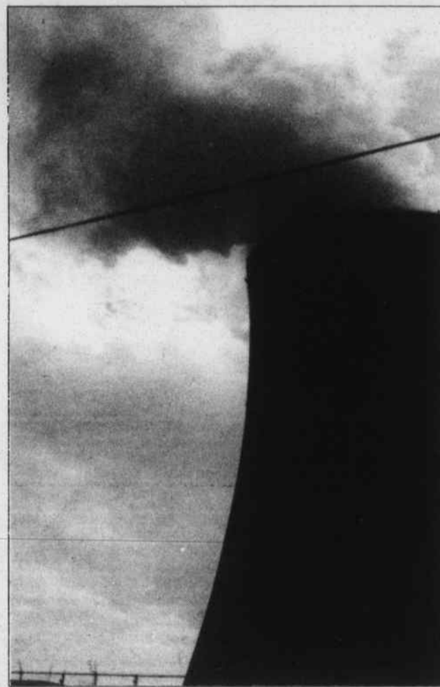
A Susquehanna nuclear power plant cooling tower
