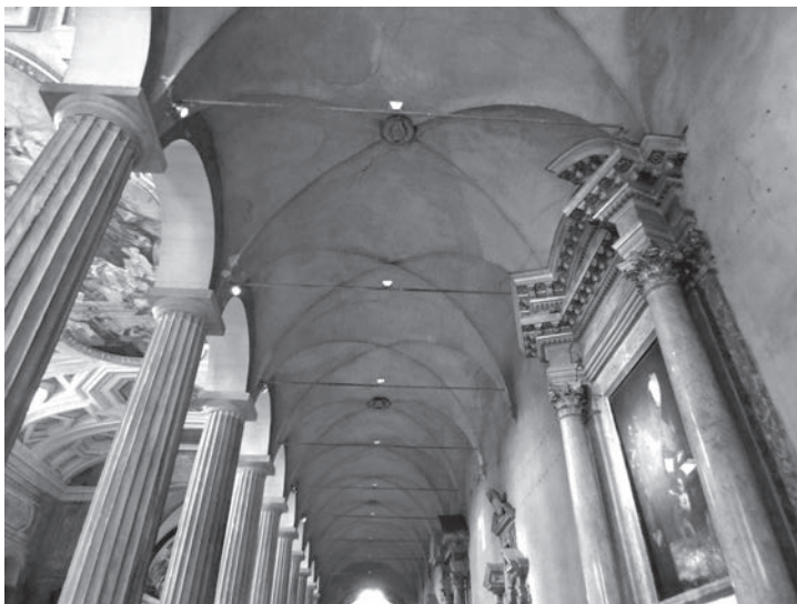
Fig. 18. San Pietro in Vincoli, Rome, aisle vault.
