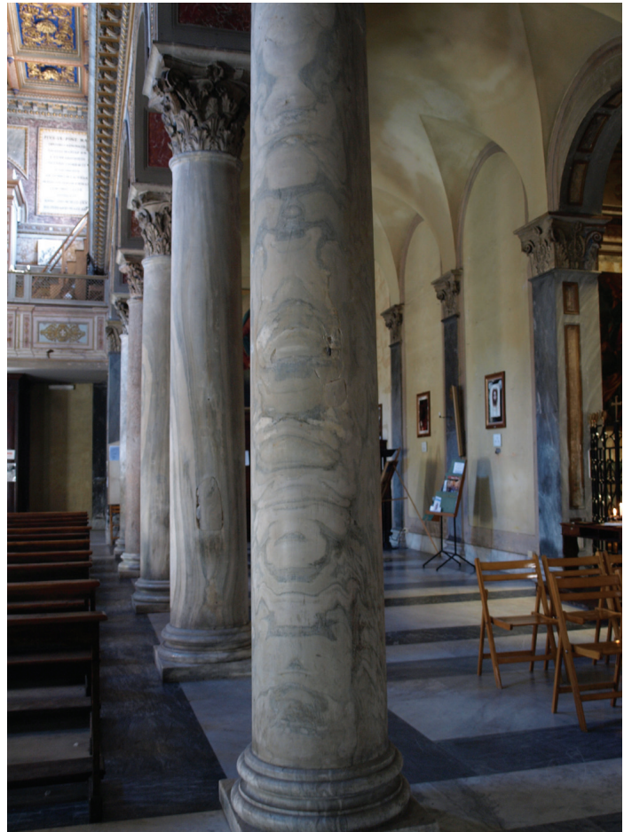
Fig. 14. Rome, San Nicola in Carcere, cipollino shafts in the south colonnade (photo: Kinney)
