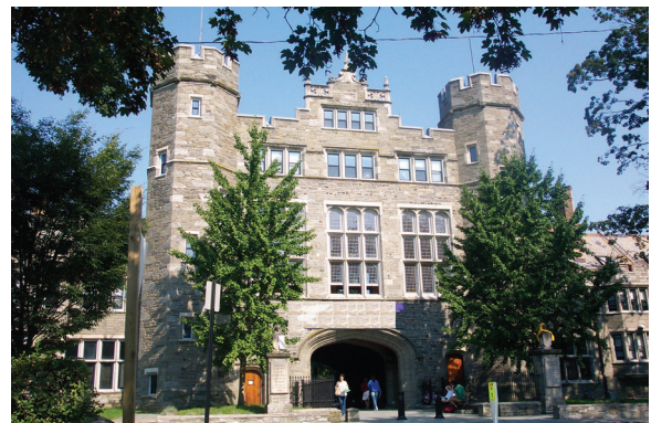
McBride Arch at Pembroke Hall
