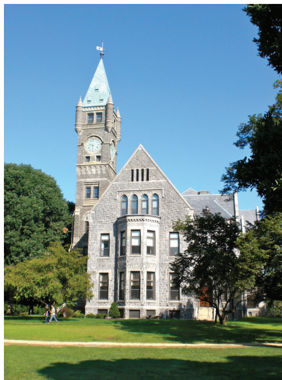
Taylor Hall's exterior renovations were completed this summer.
