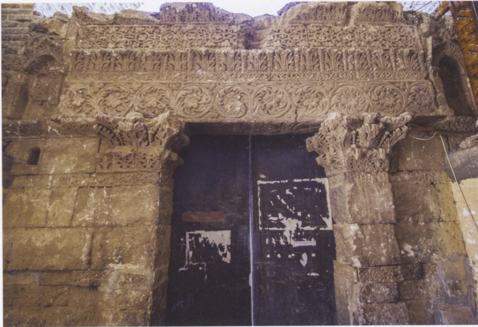
7.12 The southern portal, external facade.
