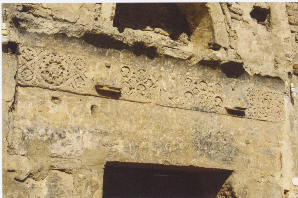
7.15 Detail of the internal facade of the northern portal.
